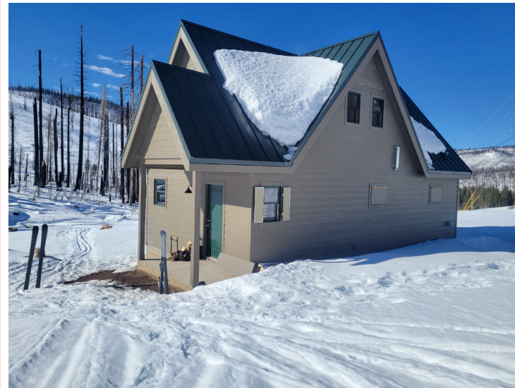
First Caldor Cabin Rebuilt - Finished, Jan '26
