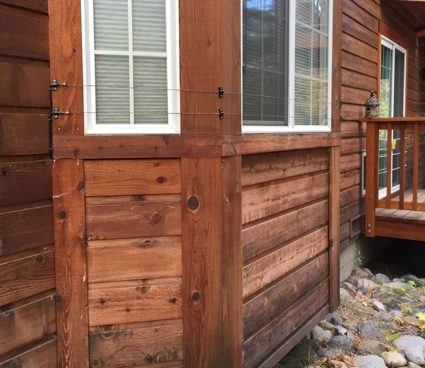
Electric fencing along windows
